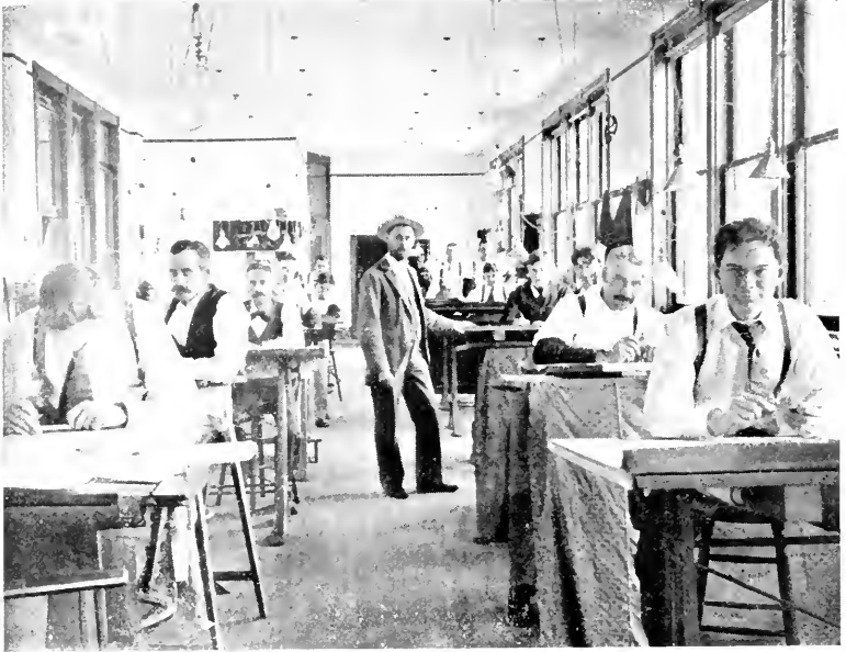
DRAFTING ROOM, GATES IRON WORKS
